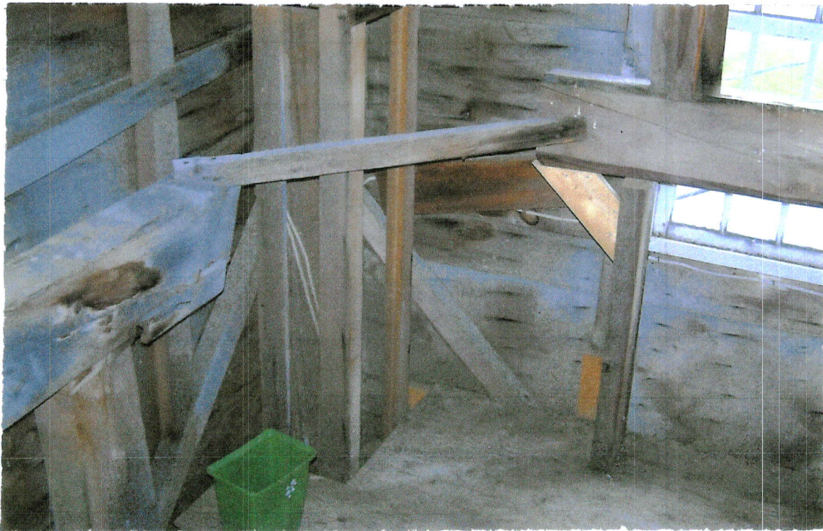
Missing 6x12" supports to lower cupola columns due to 1893 clock installation.
