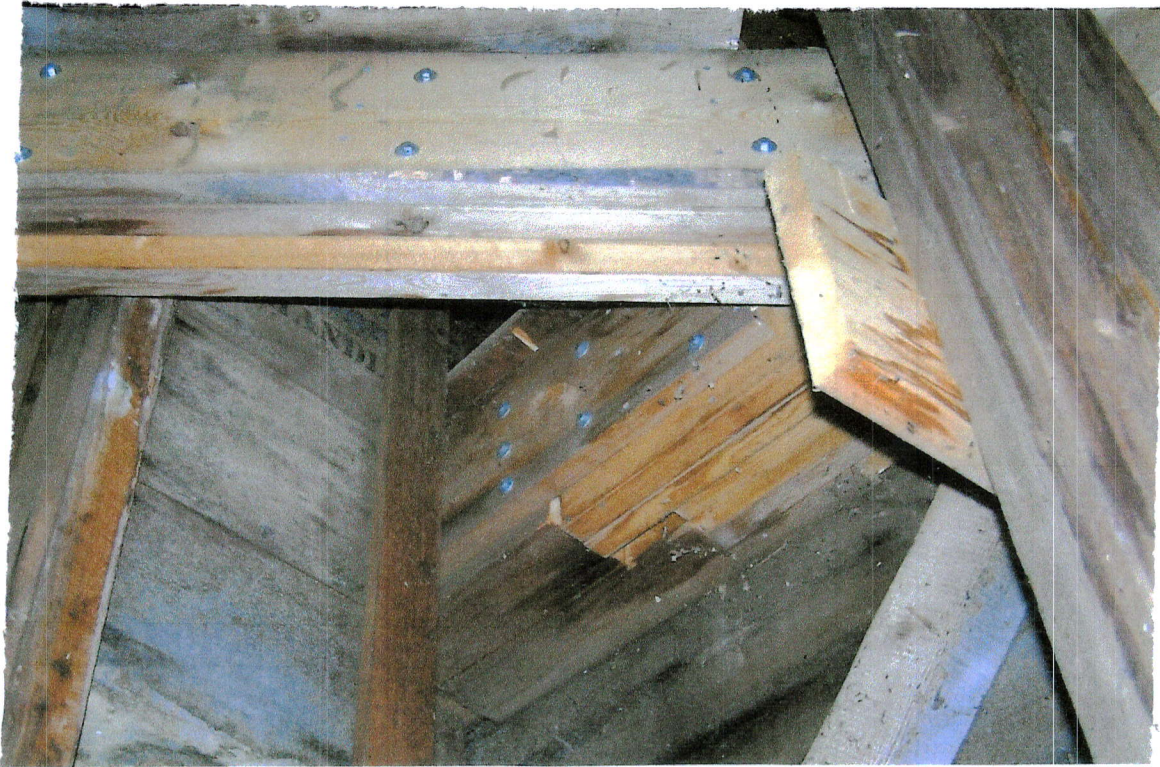
Repair beneath East clock room floor needing replacement. Provides little or no actual support to the structure.
