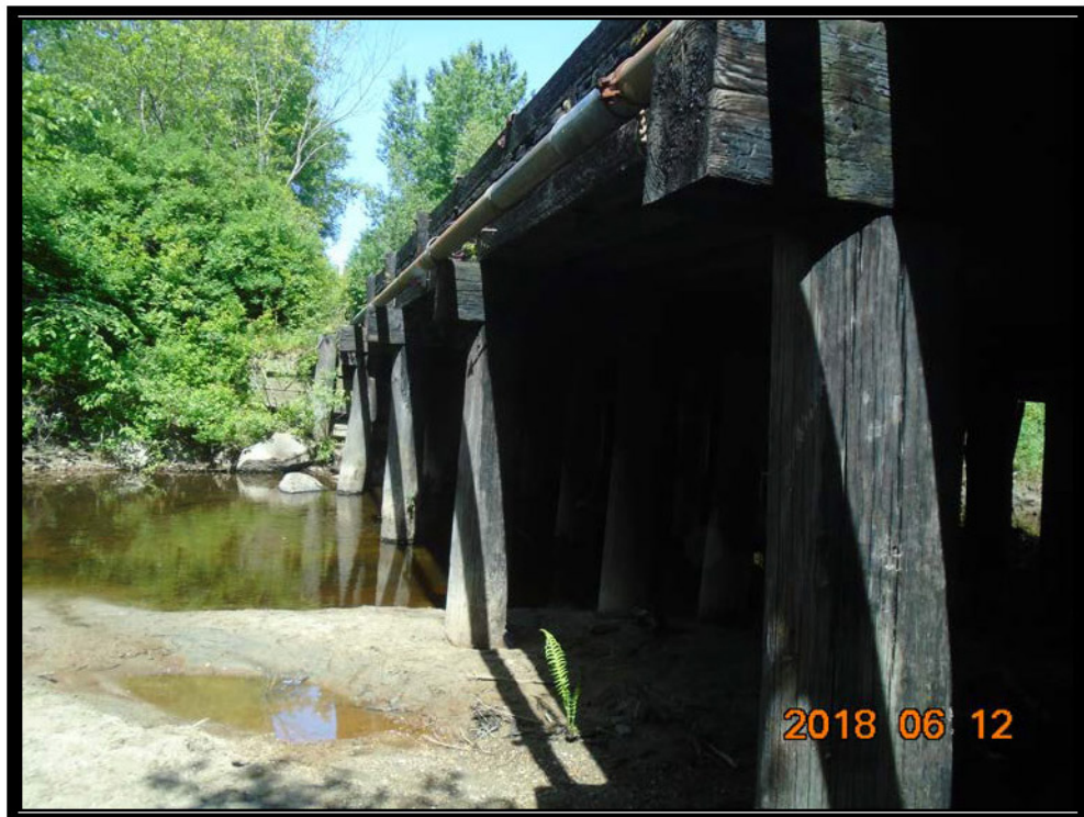
Photo 7: View of downstream side of U.T.
