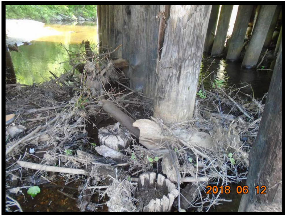
Photo 8: View of debris around piles of U.T.
