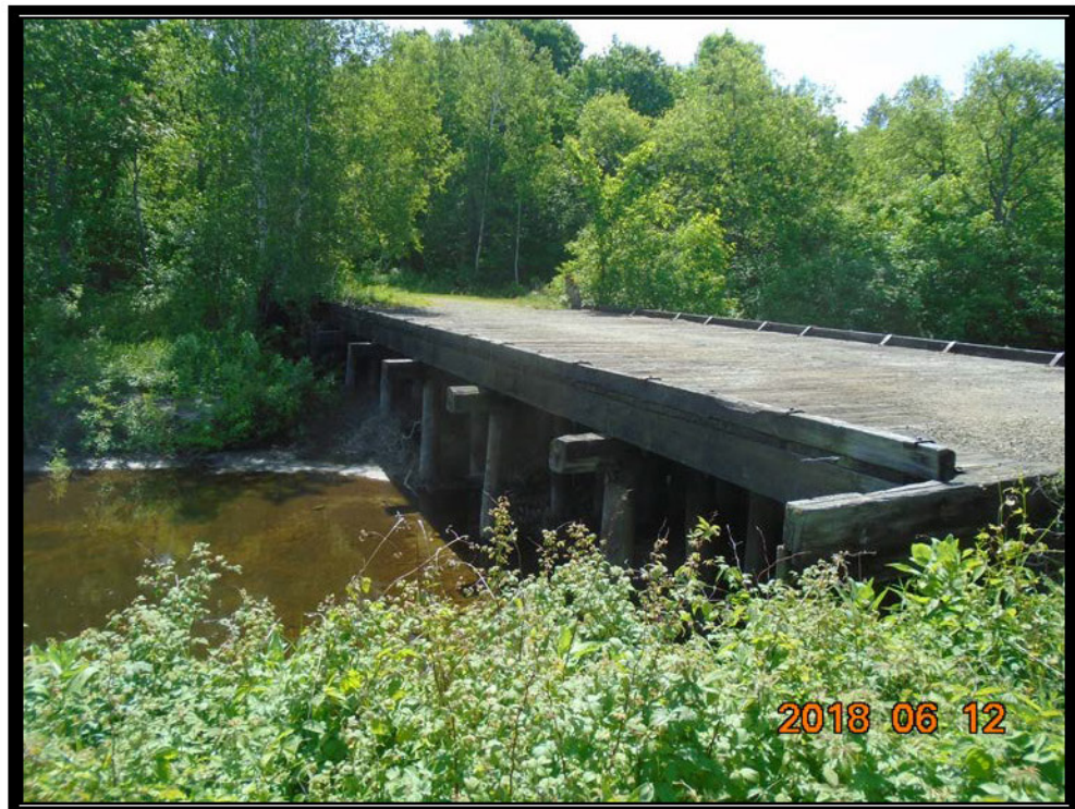
Photo 1: Looking at upstream side of Upper Trestle (U.T).
