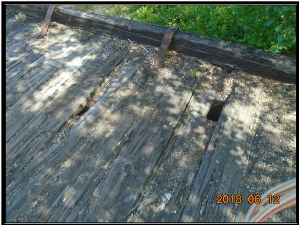
Photo 6: Looking at deck planking on U.T.
