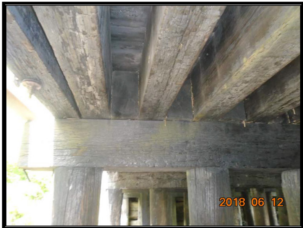
Photo 5: Looking at charred deck beams of U.T.
