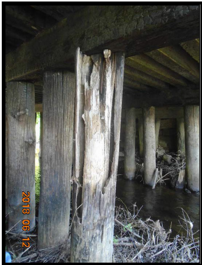
Photo 3: View of rotten pile beneath U.T.
