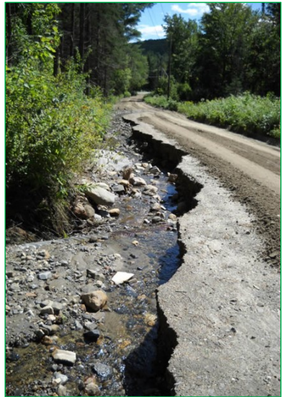
Cider Mill Road; Tropical Storm Irene Photo Credit: Town of Canaan; Emergency Webpage
